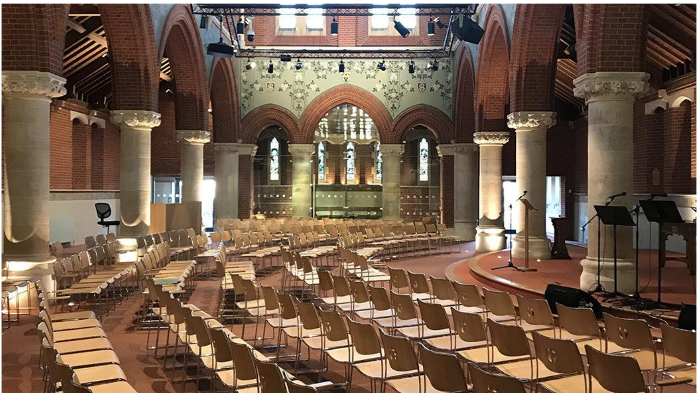
The completed conversion of St Paul's
